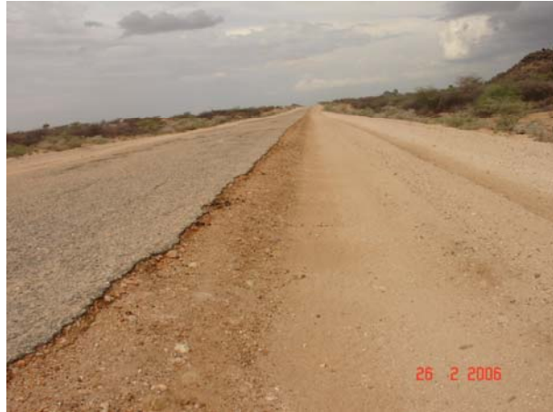
Sections of the badly deteriorated road surfacing and shoulders (left) and other sections of the same with much of the pavement structure still being intact and the graded shoulders providing an alternative roadway (right).
