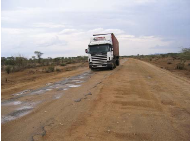
Sections of the badly deteriorated road surfacing and shoulders (left) and other sections of the same with much of the pavement structure still being intact and the graded shoulders providing an alternative roadway (right).
