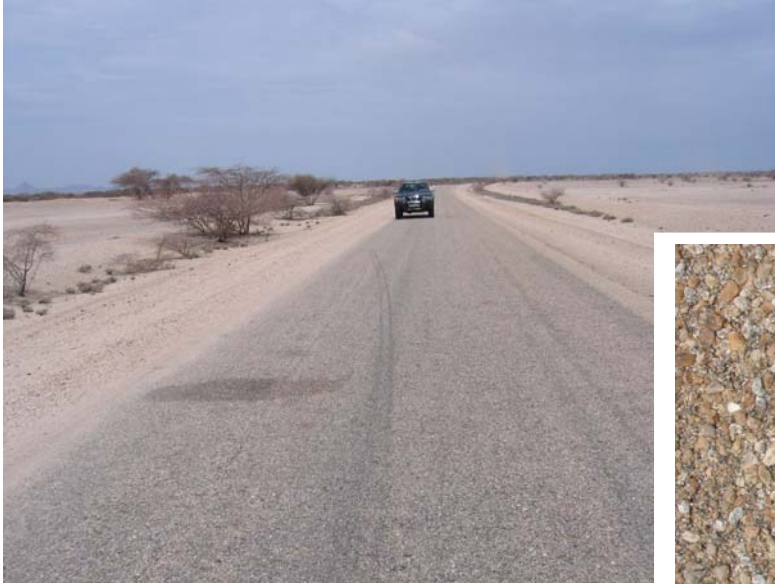
The Lodwar-Kalokol road looking towards Kalokol and showing the excellent condition of the pavement and surfacing after more than 20 years in service with practically no maintenance.
