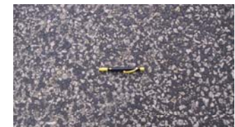
Road C 106 junction A 14. Double Otta seal using crushed coral stone.
