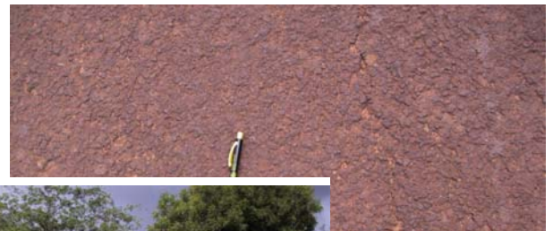
Road C 106 junction A 14. Double Otta seal using crushed coral stone.
