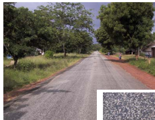
Kwale trial, "as dug" laterite as Otta Seal
